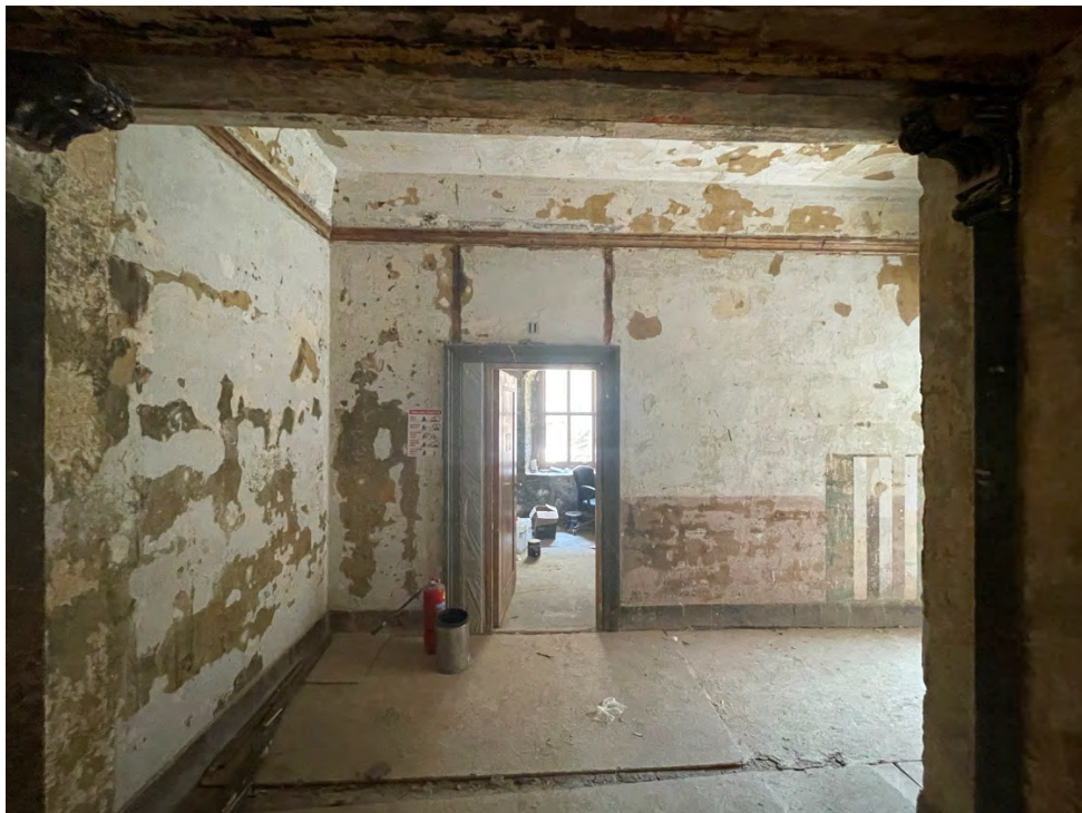
Figure 117: Room 11 (211), on the second floor. Often rented together with the adjacent room 12. The room number, "11," was recently revealed on the wall layer.
