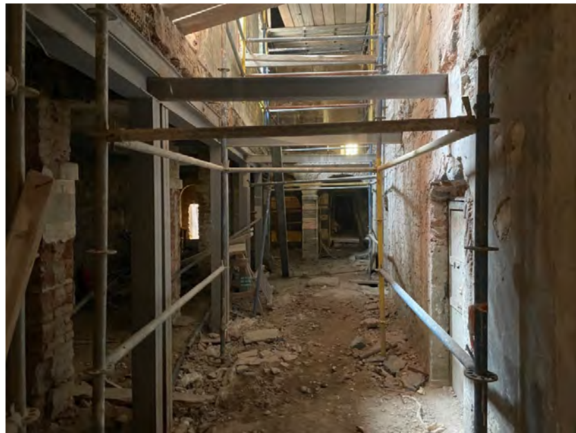
Figure 113: G18 in HC, accessible from G17. The ongoing resoration project recently removed the upper floor's slab. Source: Photograph by the author.
