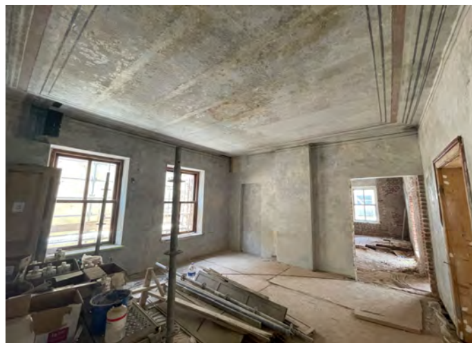
Figure 63: Room 304 on the third floor. Source: Photograph by the author.
