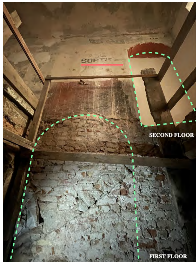
Figure 37: The blocked gates on the first floor and second floors. The exit sign “ sortie ” points to the carved wall niche on the second floor. Source: Photograph and annotations by the author
