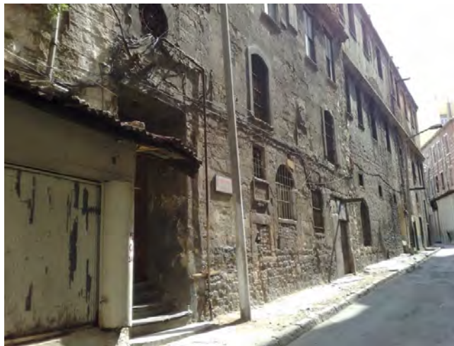
Figure 1: Saint Pierre Han, prior to the start of the ongoing restoration project in the early 2000s.
