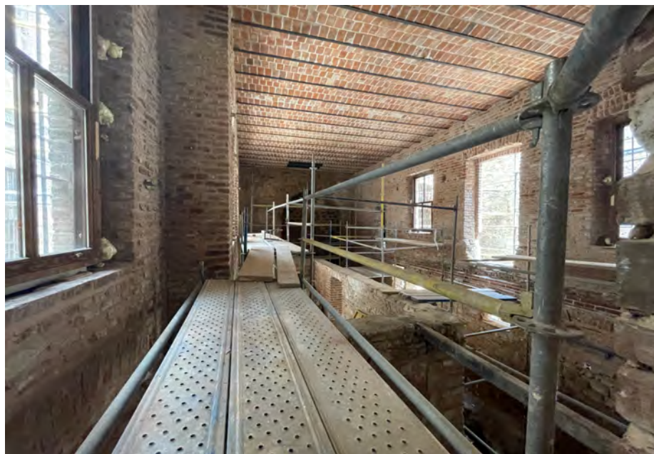
Figure 77: The area defined as HE block. The upper slab was recently removed during the ongoing restoration project, the below units are 108 and 109 of the first floor diagram. Source: Photograph by the author.
