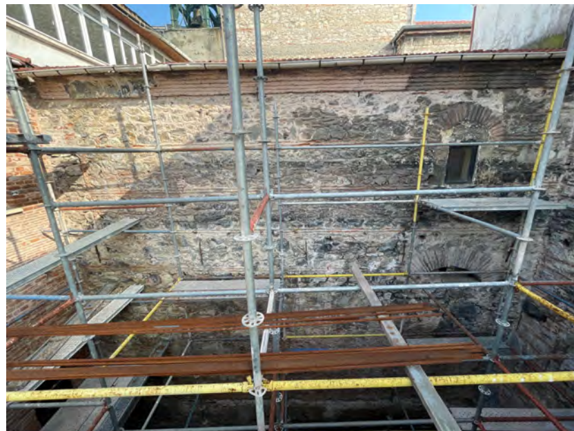
Figure 40: The bricked gates, from the han's third floor balcony (C34). Source: Photograph by the author
