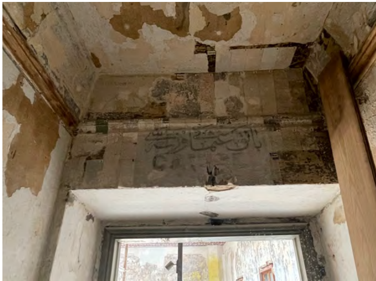
Figure 59: The entrance of room 12 (212) marks that the Imperial Ottoman Bank used this space. Later Caisse des Petits Prêts ( Dersaadet Küçük İstikrazat Sandığı ) also operated in this room.
