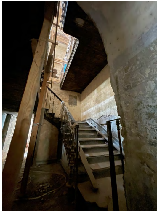
Figure 119: The wooden staircase (S5) leading to the third floor. Source: Photograph by the author.
