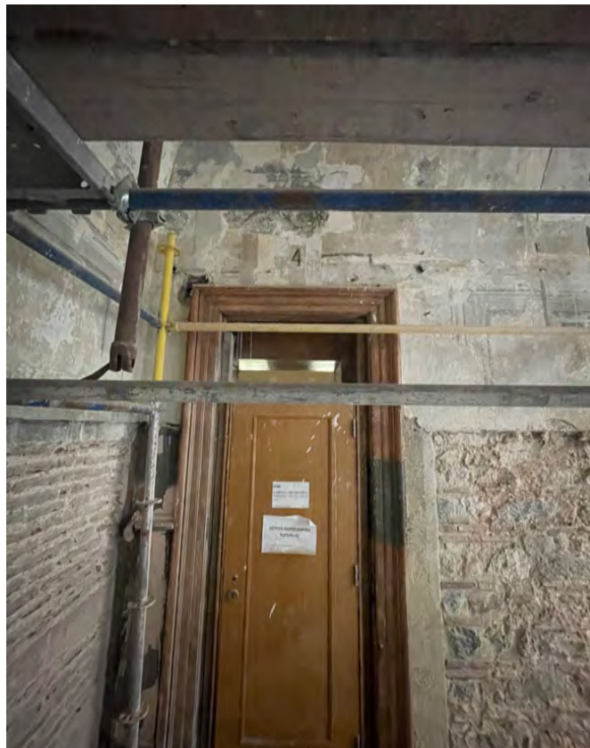
Figure 53: Room 4 (204), opening to the hall (203) on the second floor. Source: Photograph by the author.
