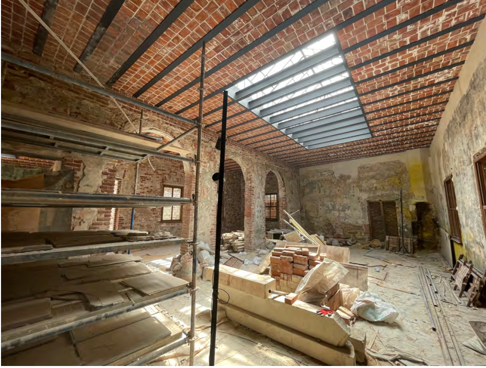
Figure 118: Interior of room 12 (212), served the Imperial Ottoman Bank's cashier hall, and later Dersaadet Küçük İstikrazat Sandığı . The ceiling and skylight were recently restored based on original form. The terrace is located on top. Source: Photograph by the author.
