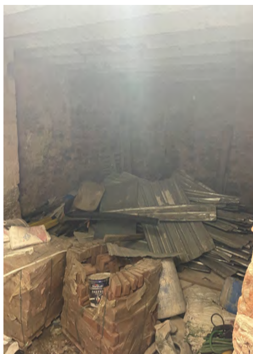
Figure 60: G02 on the ground floor, one of the designated storage spaces in Saint Pierre Han.
