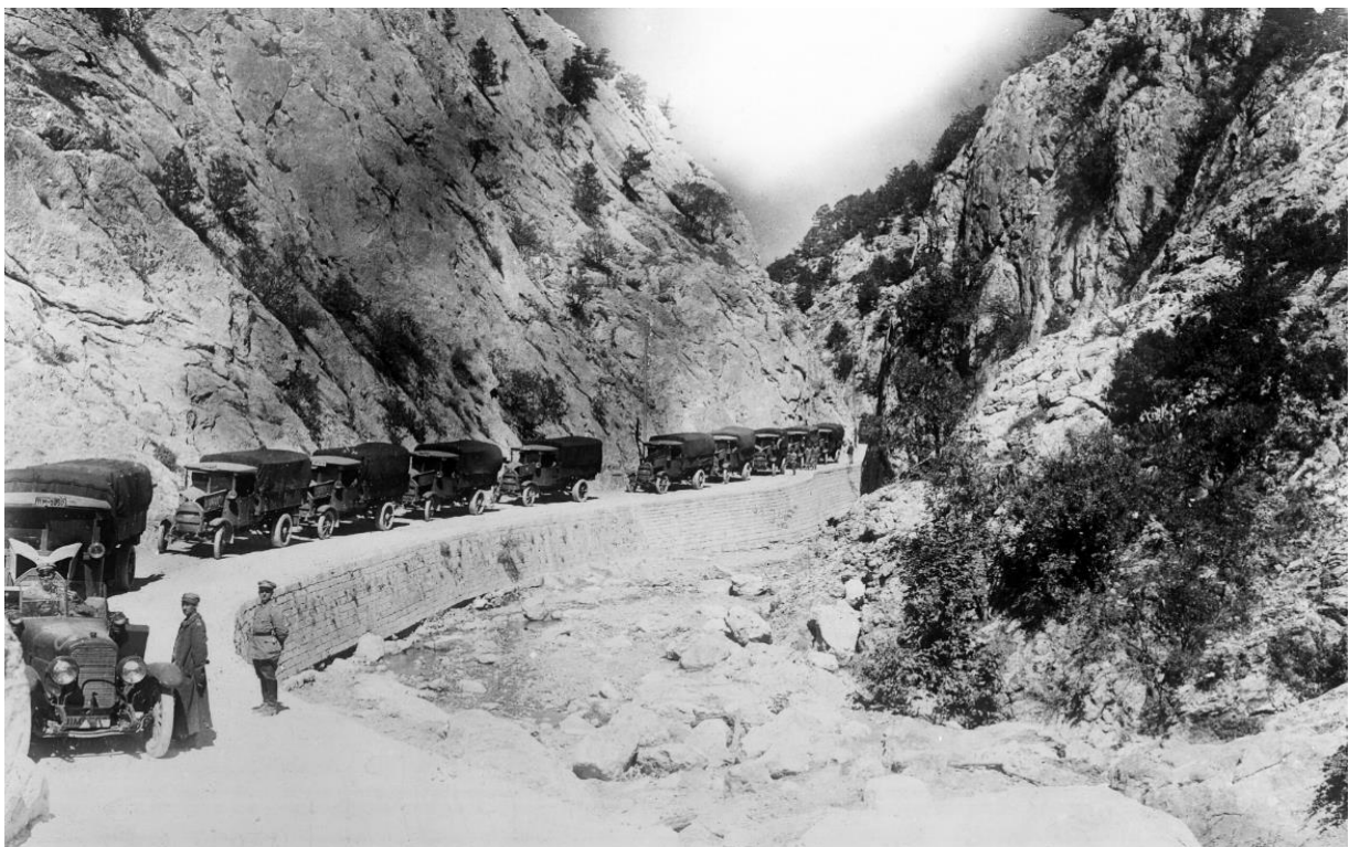
The road through the Taurus Mountains, constructed by POWs.
