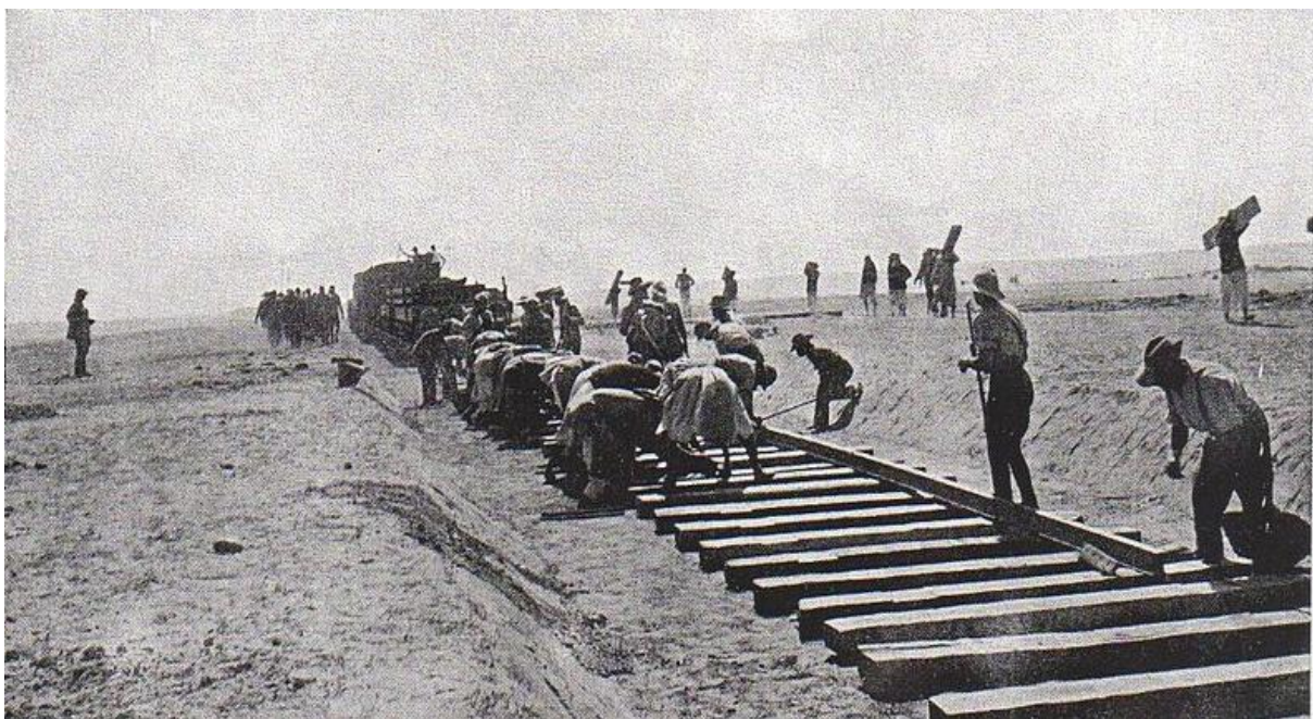
Building the Sinai Railway
