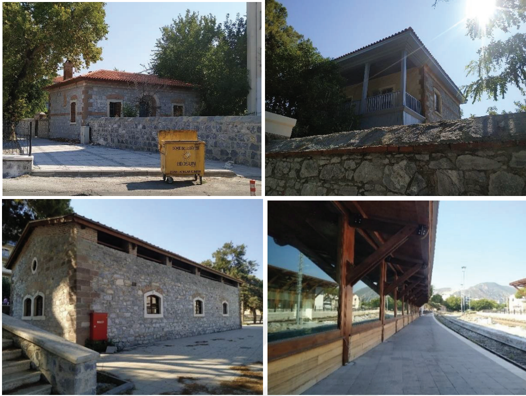
Figure 84. Guest houses of the Söke station and warehouses from Söke station, recently renovated by the author, 2019
