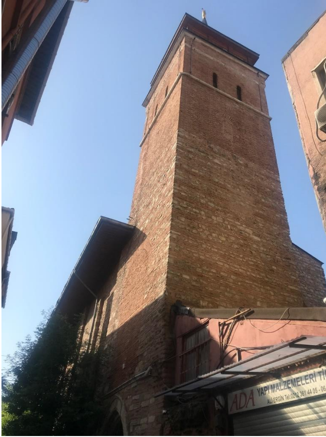
Fig. 41: Arap Camii/San Domenico and minaret/belfry. Photographed by author 2021.
