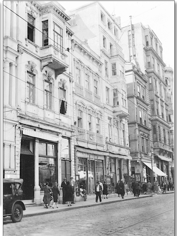
Building on the left is thought to be Nikitiz Han, Grand Rue de Pera, where Elsie and Arthur Leavitt had their first apartment. Arthur Baker's car is apparently parked out front. Two doors down to the right is the Baker shop at No. 370 Grand Rue de Pera, although George Baker's name is no longer there (c. 1912).
