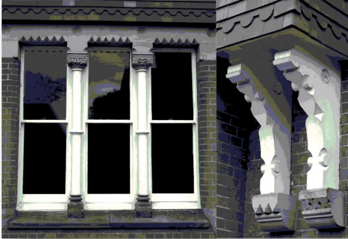
Front bay columns and stone finials
