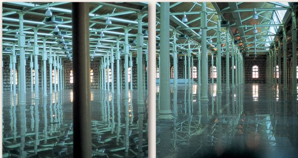
Original steel columns of the Feshane factory building, supplied around 1856 by the company << Providence >>, from Marchienne in Belgium.
