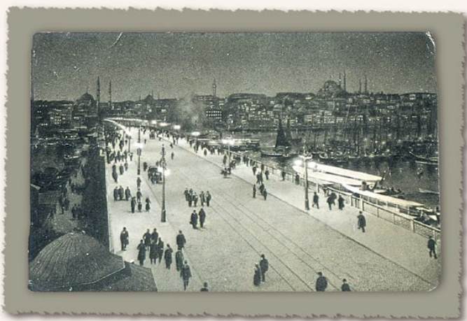
First lanterns on the Galata Bridge, as part of the network established by << Gaz de Stamboul >>. Collection S. Kayserilioglu
