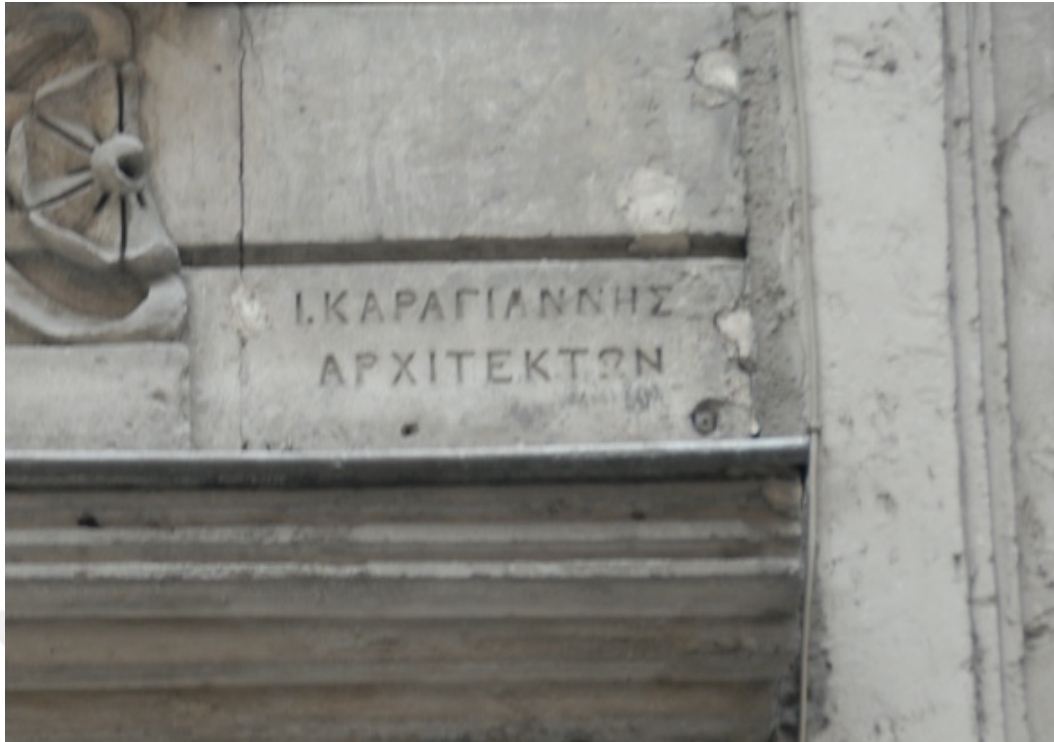
Figure 86: Ioannis Karayannis, Kehayioğlu Apartment – detail above the main entrance, Siraselviler Street, 1903. Photo: Merve Uca
