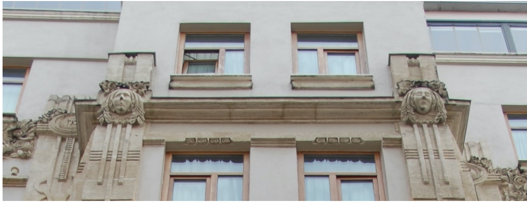
Figure 112: Yeorgios Kuluthros, Parma Apartment – detail from the façade, Meşrutiyet Boulevard, early 1900s. Photo: Merve Uca
