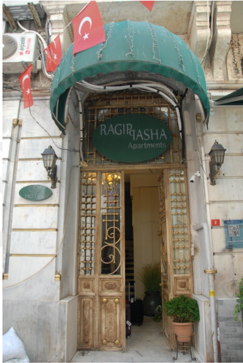
Figure 94: Aram & Isaac Caracach, Ragıp Pasha Apartment – door detail, Grand Rue de Péra, early 1900s. Photo: Merve Uca
