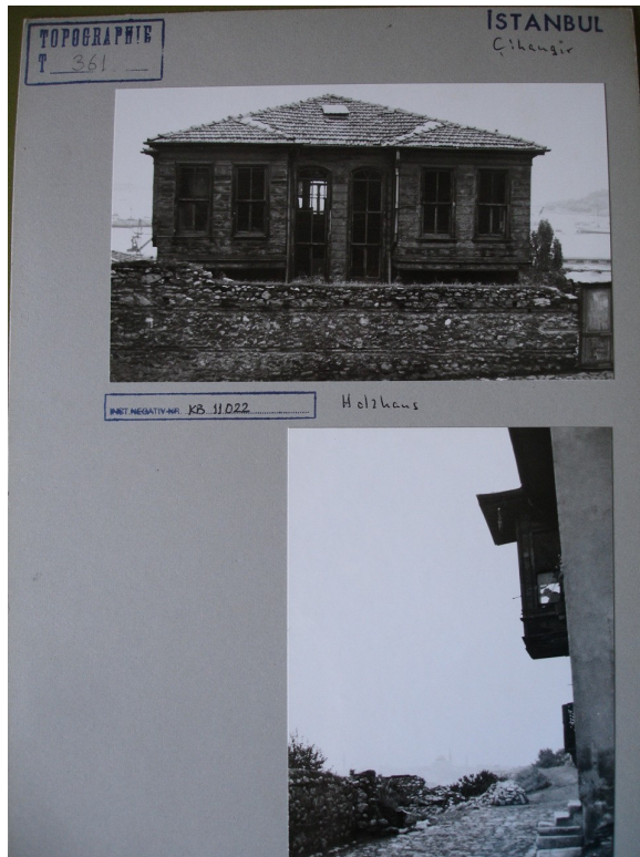
Fig. 8 A decaying house in Cihangir
