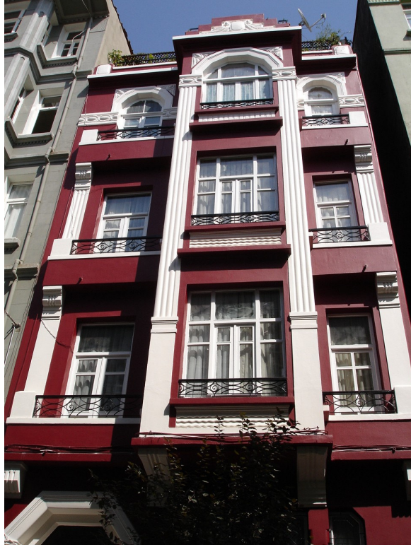
Fig. 14 A renovated apartment building in Cihangir, photograph taken by the author, 2006
