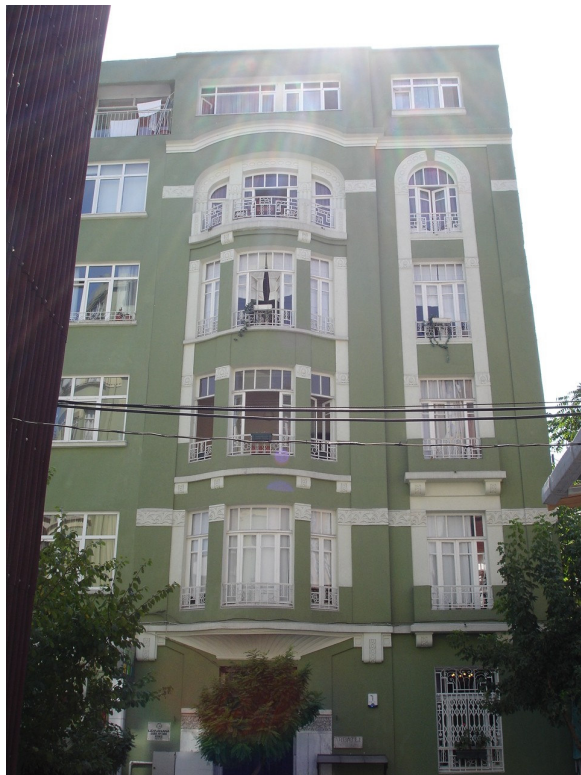
Fig. 25 Apartment building in Akarsu Street, photograph taken by the author, 2006
