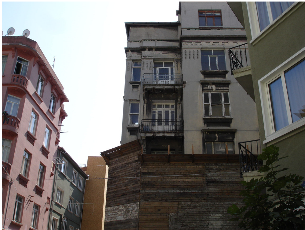
Fig. 17 An apartment building under renovation, photograph taken by the author, 2006
