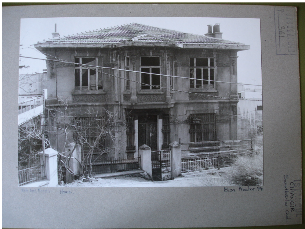
Fig. 7 An old abandoned house in Cihangir, 1994
