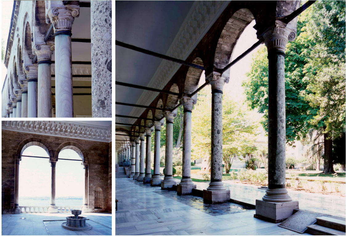
Fig. 16. Courtyard arcade and loggia with fountain at the Inner Treasury of the Topkapı Palace. (Photos: courtesy of Hadiye Cangökçe)
