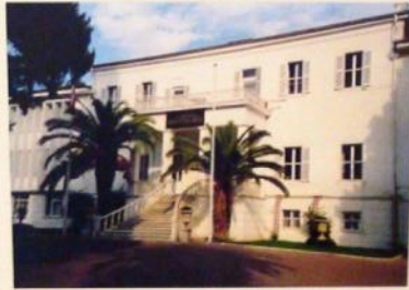
The Big House home of James John Whittall (extended and currently used as the residence of the Dean of Ege University)
