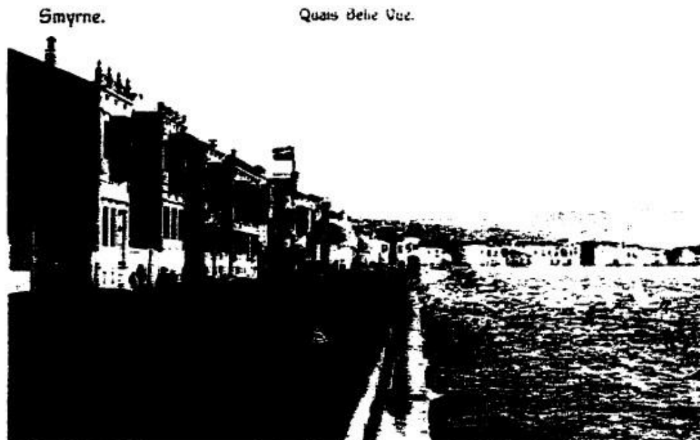
Figure 35: View of the new quay (Suna Inan Kır aç Research Institute on Mediterranean Civilizations).
