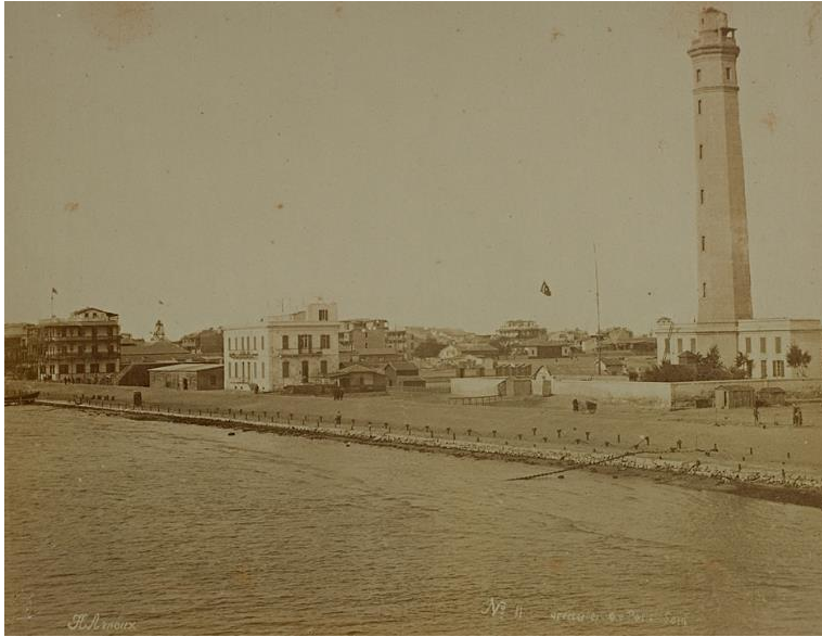
Figure 8 Port Said Lighthouse in the entrance of Suez Canal 199
