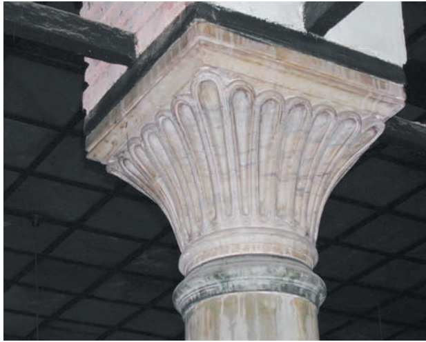
Fig. 15. A capital in the revak (arcade) of the Madrasa of Seyid Ahmed Pasha.
