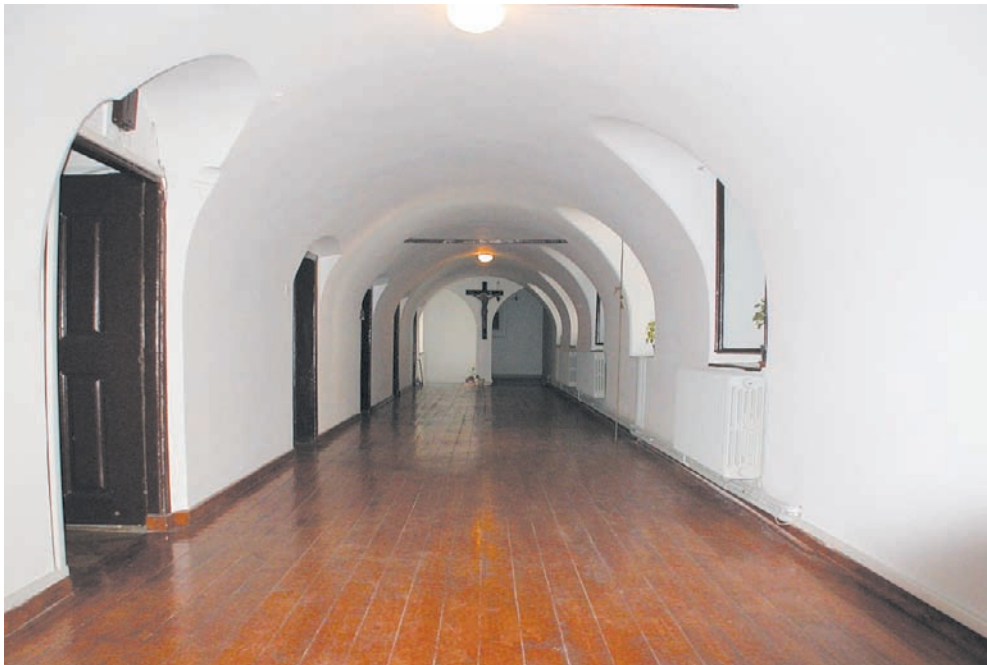
Fig. 10. Santa Maria Draperis, corridor in the upper story of the convent.
