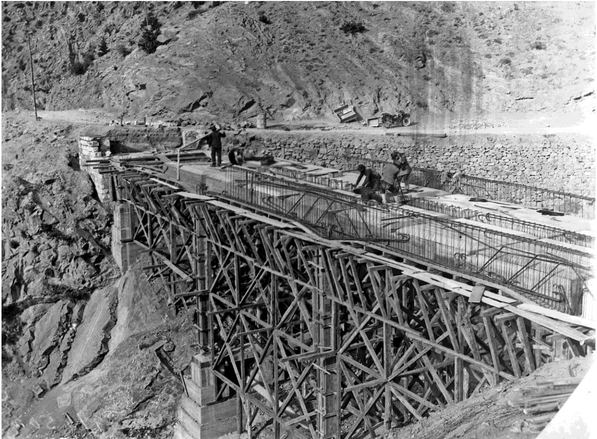
Construction of one of the many bridges.
